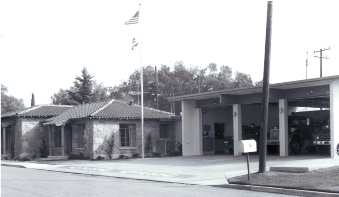
Station 45, Simi's first fire station building constructed in 1937 with engine room added in 1964.
