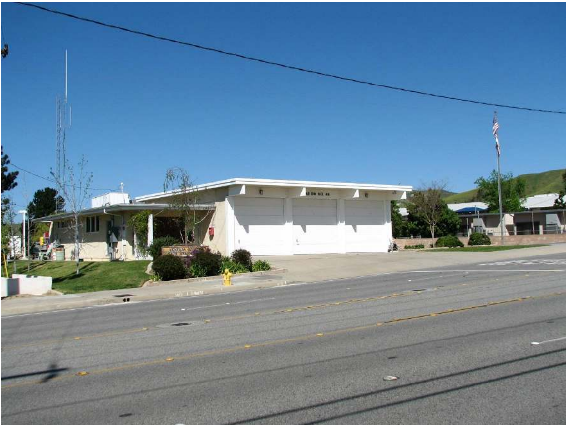
S-46 prior to 2013 remodel.
